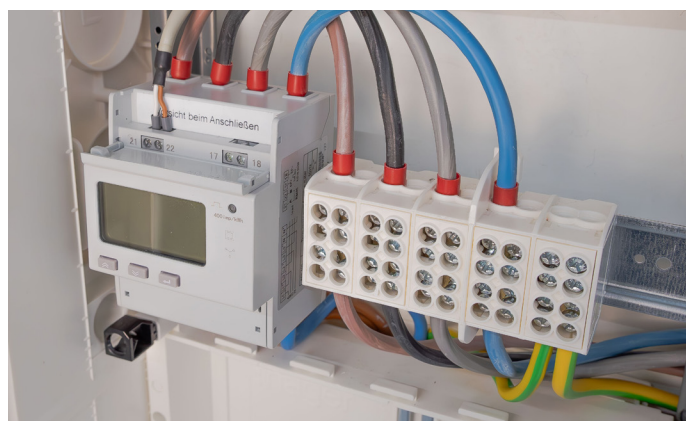
Fig. 36 ADL400 correctly connected
